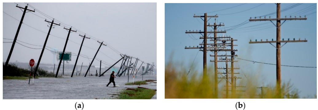
Figure 7. (a) Electric pole falls due to floods [61]. (b) Wooden electric pole [62].
